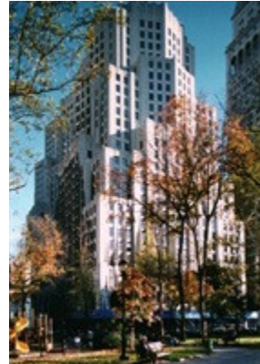
The Metropolitan Life Bldg. in Manhattan, one of several buildings using energy-efficient ice-cooled air-conditioning systems.
